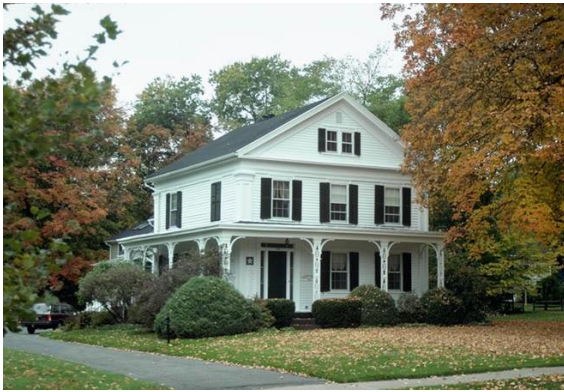
31.1 Proper eave detailing is not difficult or cost prohibitive, it just takes a little time and will convey a sense of true craftsmanship .
