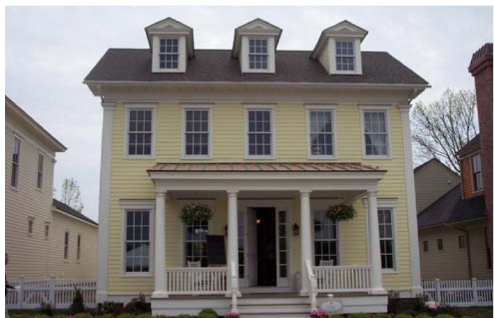
40.5 Step the dormer back from the facade of the house so that they are in different planes. Keep the dormer beneath the ridgeline to maintain proper hierarchy.
