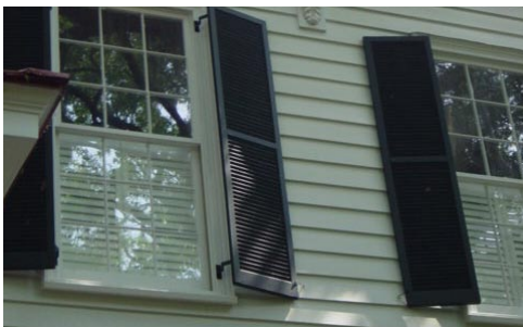
35.3 Shutters should be operable, or appear operable, and be sized to fit the window when closed.
