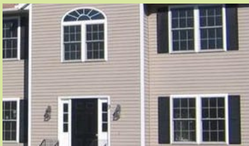
35.4 The shutters on the building above would cover only half of the necessary opening if they were ever closed.
