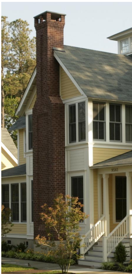
42.1 Continue chimneys down to the ground. They require visual and structural support at the foundation. Build chimneys of masonry or, at the least, non-flammable materials. Detail the chimney cap in a simple, easy to build manner.
