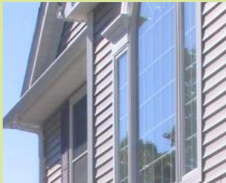
35.2 Windows with applied muntins on the exterior face of the lite, or embedded within the double glazing lack the depth and interest that true muntins create.
