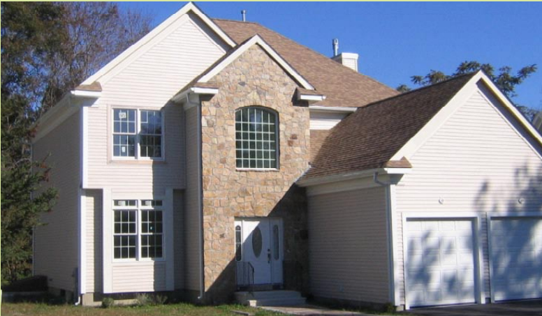
29.2 Don't - The examples above illustrate volumes that have stone applied to a single face with clapboards returning on either side. The resulting effect is that of a Hollywood stage set, revealing the use of stone as an applied surface. Such treatment of the material is wholly inappropriate for the weight and mass of the material.
