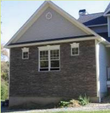
29.2 Don't - The examples above illustrate volumes that have stone applied to a single face with clapboards returning on either side. The resulting effect is that of a Hollywood stage set, revealing the use of stone as an applied surface. Such treatment of the material is wholly inappropriate for the weight and mass of the material.
