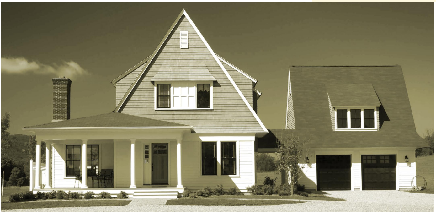
28.4 The garage is deferential to the main house by having a lower roof spring line than that of the main house. However, the two structures share similar materials and proportions, creating an aesthetic harmony among all parts.
