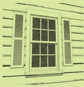
35.4 The shutters on the building above would cover only half of the necessary opening if they were ever closed.
