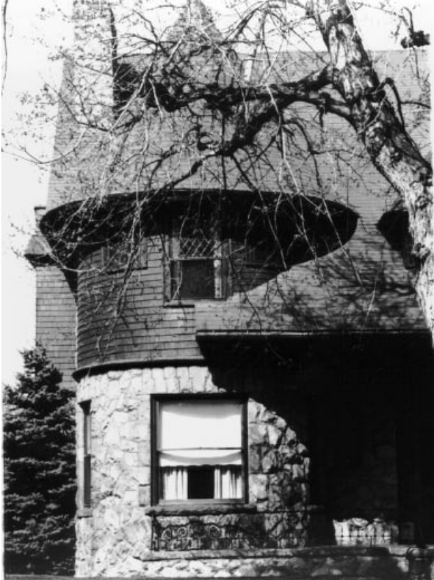
29.1 DO - The image above is a classic use of stone to form the base of a turret on a shingle style building. While the rest of the house may be shingle - the stone is used consistently to highlight the base of this volume. Stone is a visually “heavier” and a stronger material than shingle; in traditional construction, heavy materials are always used at the base to support the building above.
