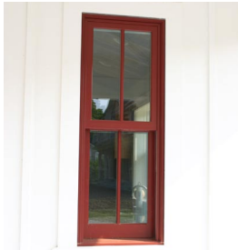
35.1 The most visually appealing and properly constructed windows have true muntins separating each window lite.
